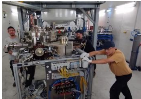
Dismantling of the PPF ( September 2023 )
