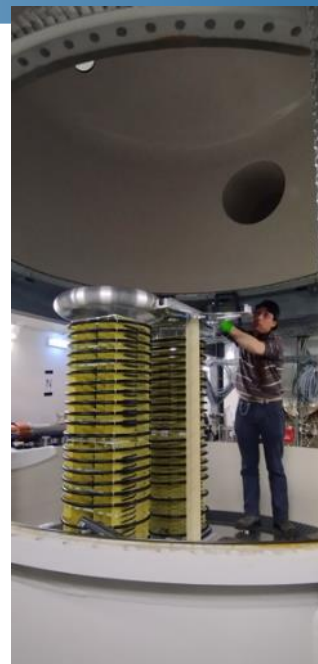
Dismantling of the HV Columns tanks Dismantling of the platform done by Baumann ( November 2023 )
