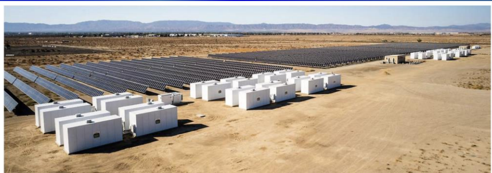
Figure 7: A single 25 MWh energy storage unit (white containers) built from used electric car batteries, deployed for a PV energy plant in Lancaster, CA (south of Los Angeles, US) put in operate by B2U Storage Solutions in early 2023. Capacities of new systems are increasing fast. A 260 MWh 25 is by now being commissioned and today's largest systems in the range of 1 400 MWh are being extended to 3 000 MWh 26 .
