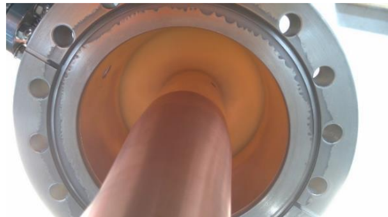
1#: Window cracked due to FE (Spoke021 SCC for CADs)
