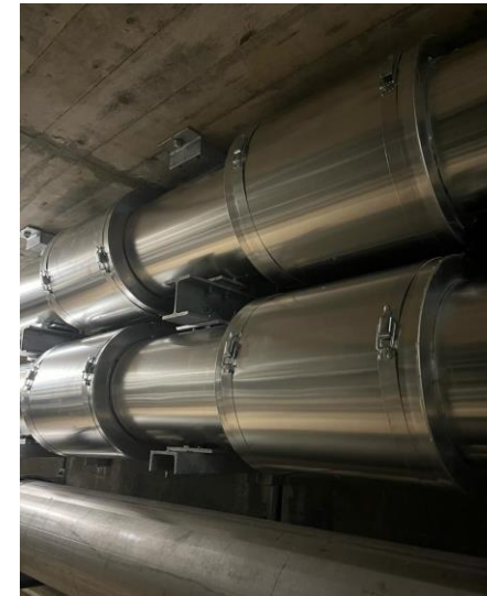
INSTALLATION OF INSULATION
