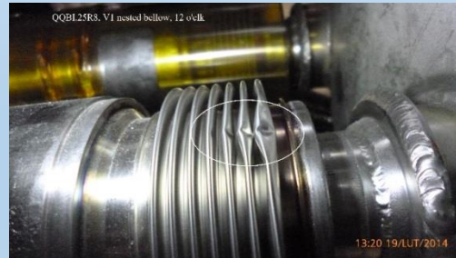
Damage disclosed during QC- ICIT TEAM
