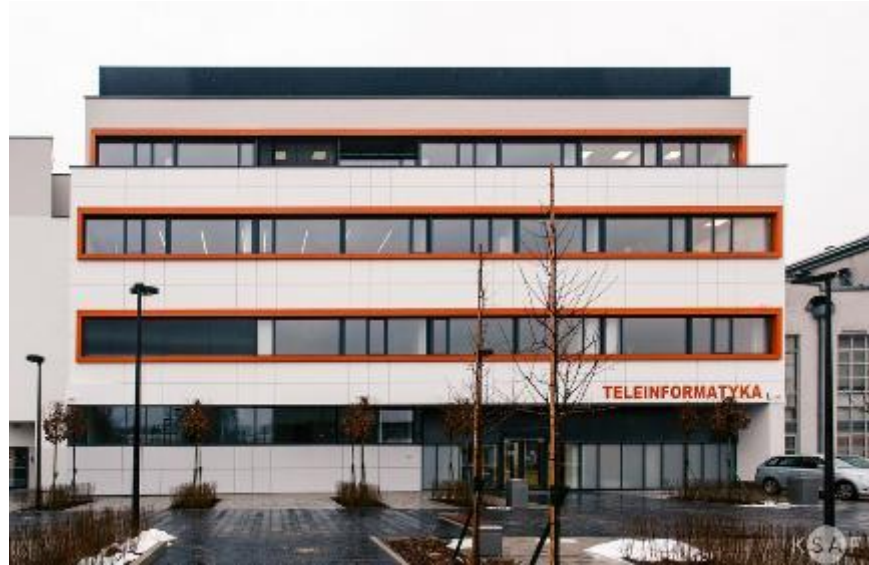
Department of Telecommunications, II
