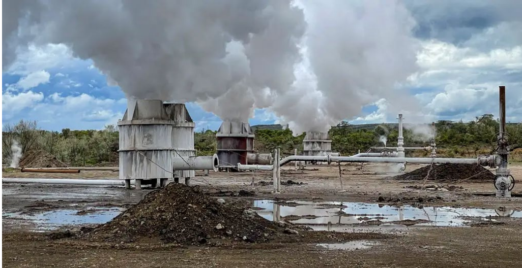
Expanding Kenya's Olkaria Geothermal Power Station
