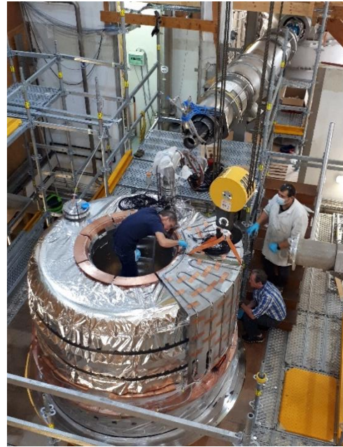
Assembly of the thermal shields
