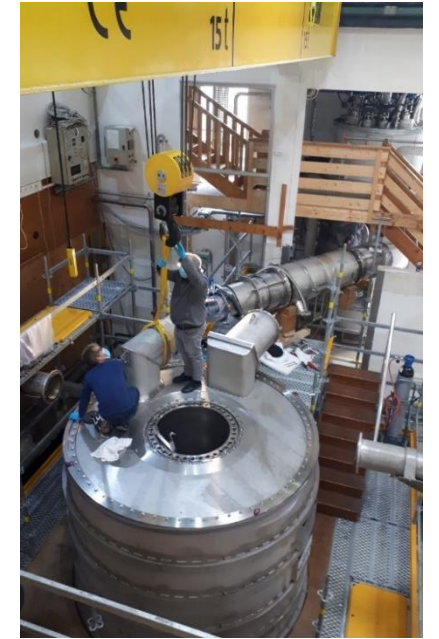
Installation of the OVC
