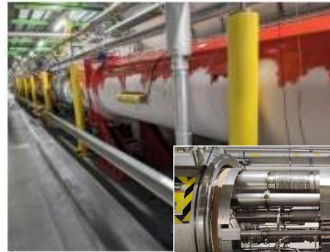
Leak on bellow of Q1-Q2 interconnect L8
