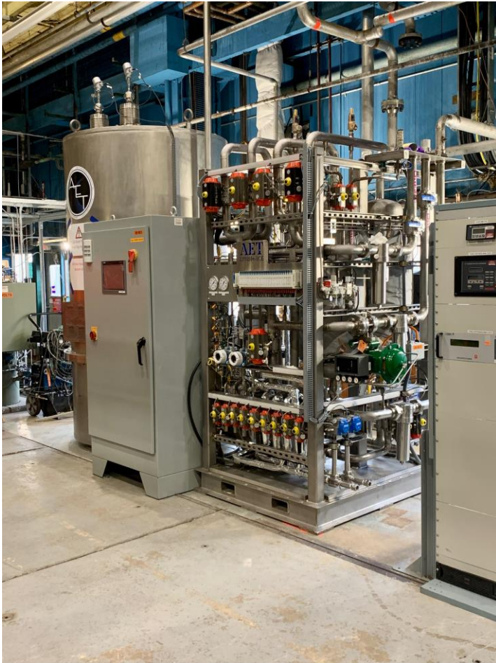
Installation of New Purifier
