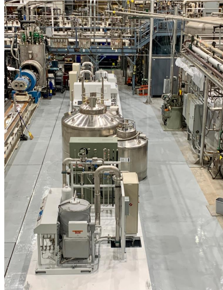
Installation of New Linde 1630 (70l/h) and 1430(40l/h)
