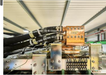
Water-cooling network and water-cooled cables
