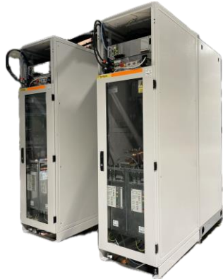
HL-LHC energy extraction systems
