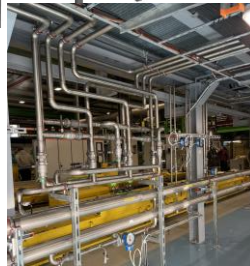
Water-cooling network and water-cooled cables
