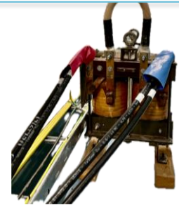
0.4 mH Inductor added for the 200 A circuit
