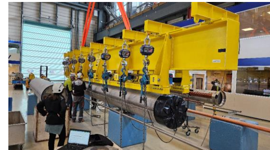
Chain hoists to adjust accurately the load for each cable when handling the cold masses replacing tensioners left/right
