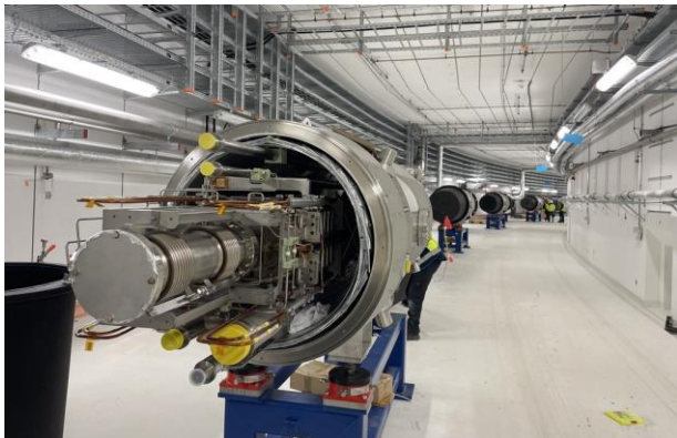
First magnet installations in tunnel
