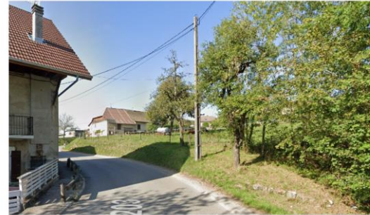
The clearance in correspondence of the curve is too small; the utility pole shall be relocated and some works on the outer side of the curve is necessary.
