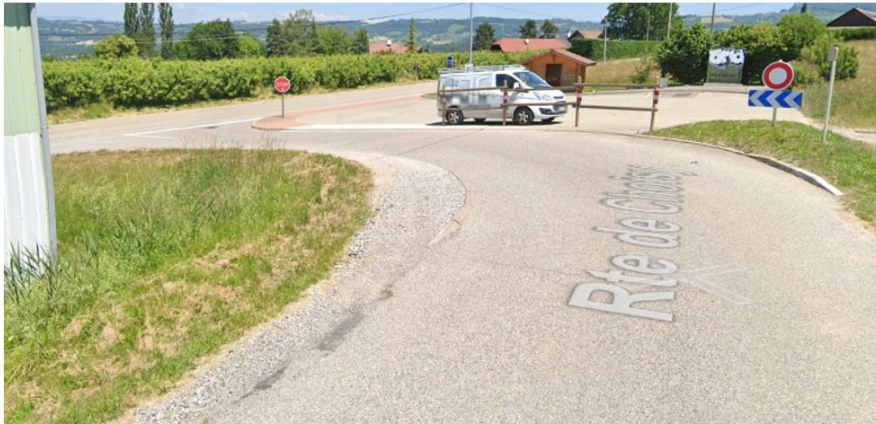
The curve at the intersection D2 – D203 is too narrow for this type of convoy. A solution would be that the convoy advances after the intersection and the tractor is switched from the front to the back of the trailer.
