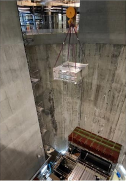
Bottom TPC installation (September 2023)
