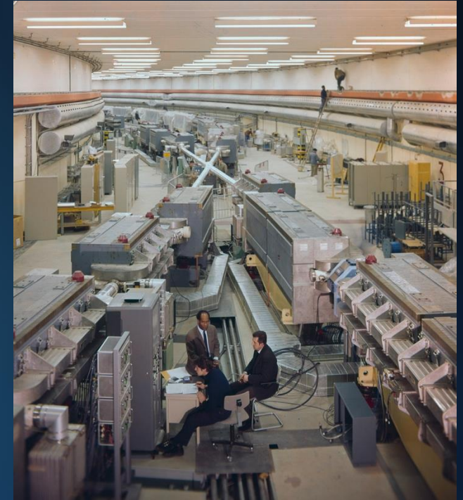
Intersecting Storage Ring
