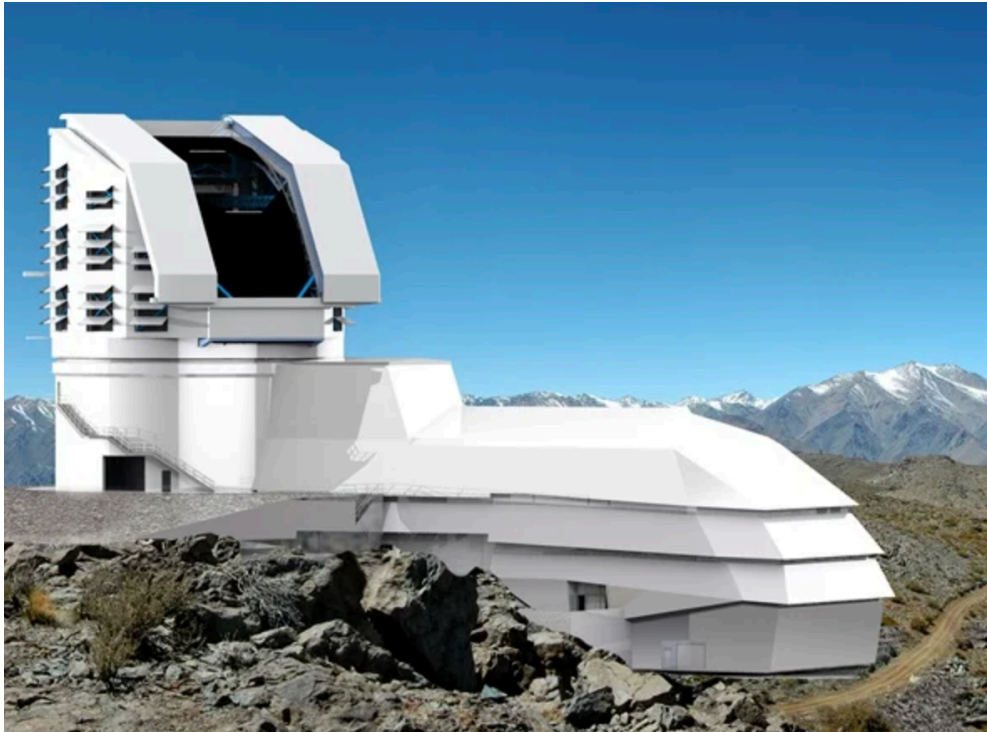
Legacy Survey of Space and Time (LSST)
