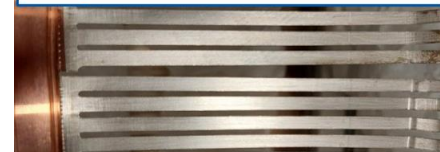
Example of damaged RF finger of A4L1 warm module
