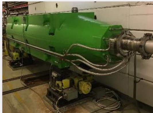
Assembly inside tunnel
