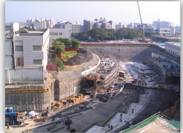
Civil works as of December 8, 2010.
