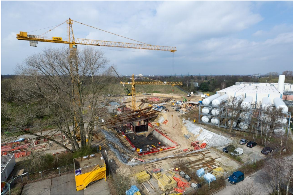
Construction of Injector Vault on DESY site; April 4, 2011
