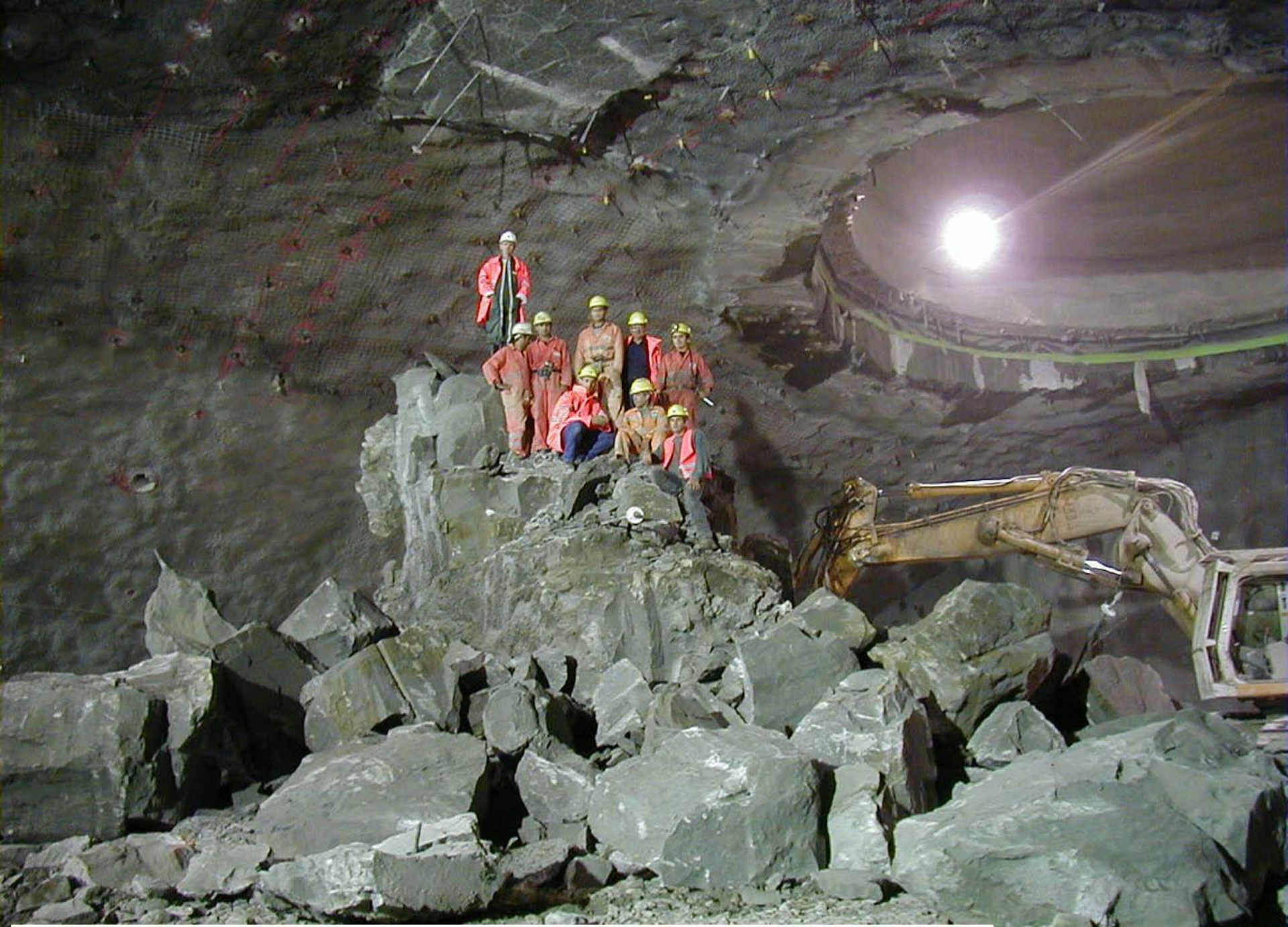
Point 1 - UX15 vault demolition of central pillar - September 20, 2000 - CERN ST-CE
