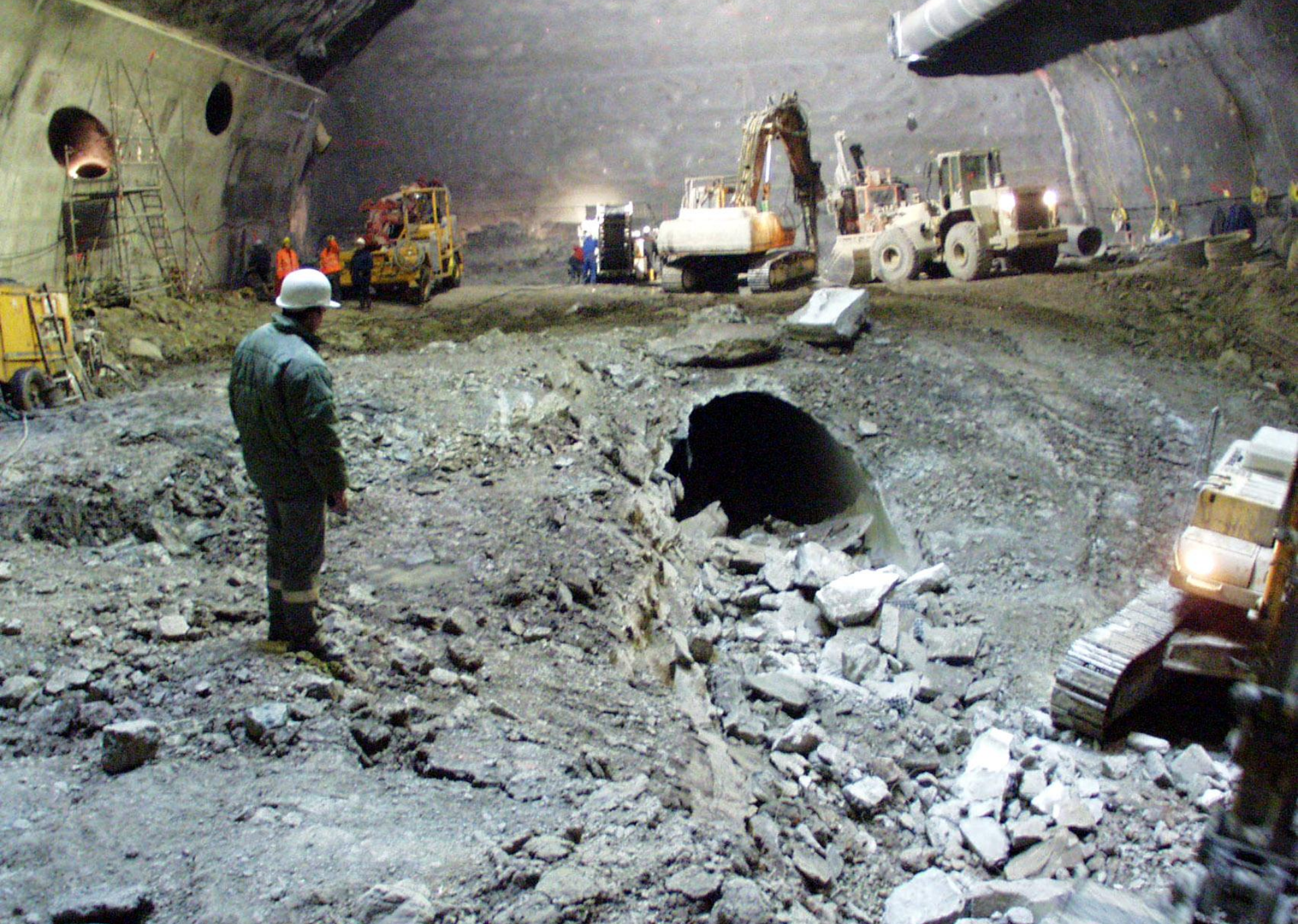
Point 5 - UXC55 cavern excavation - LEP demolition - January 23, 2002 - CERN ST-CE
