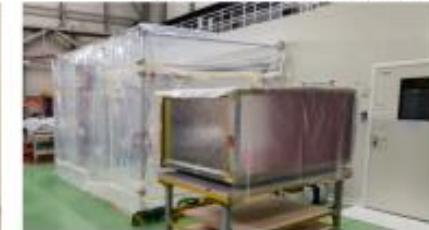
Grey tent area in front of Clean Room large entrance for enhanced clean conditions
