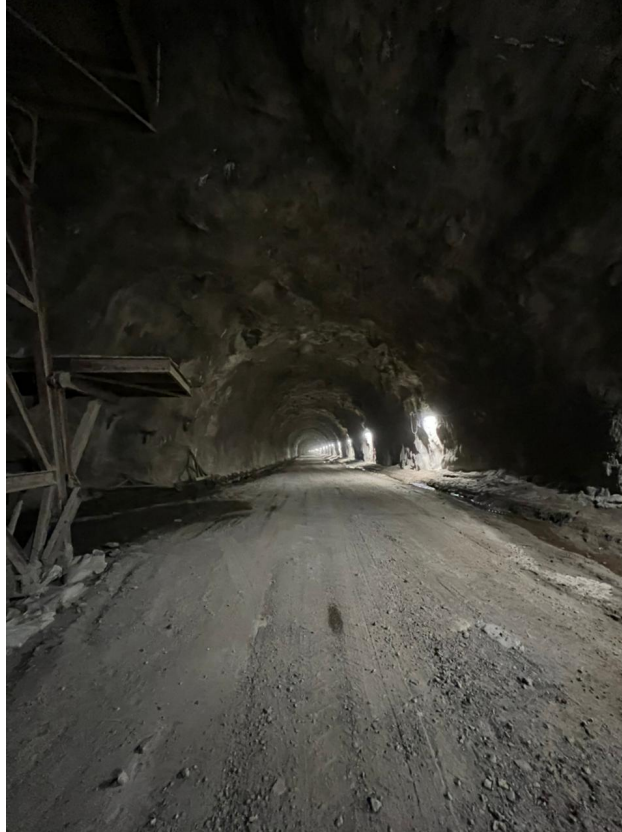
Figure 17-2. Inside the Huguenot Tunnel. Photo credit: courtesy Richard Newman/Stellenbosch University.
