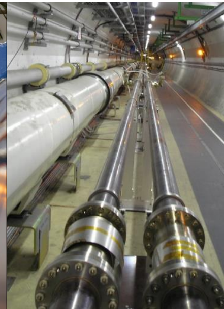
LHC Cryogenic and RT beam pipes with 1-2 \mu m-thick NEG-coating (Ti-Zr-V)
