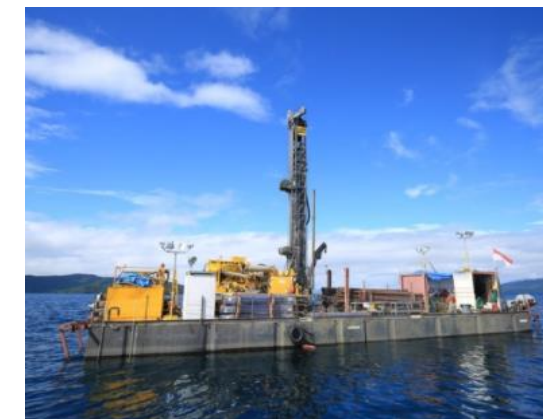
example of drilling works on a lake the lake
