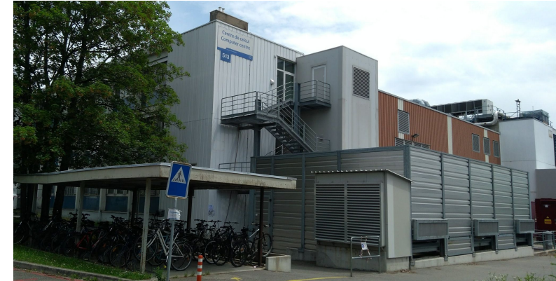
Meyrin Datacenter (MDC)
