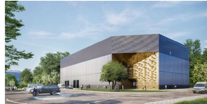
Preessin Datacenter (PDC)
