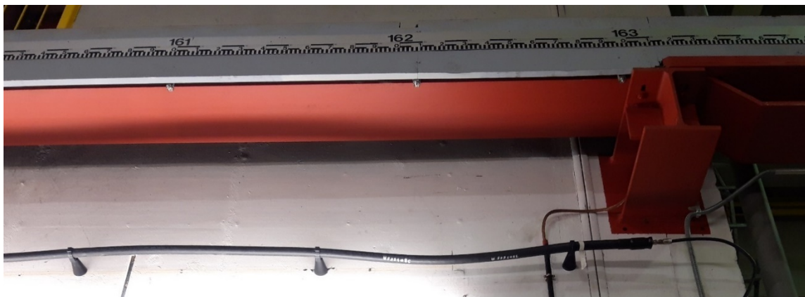
Figure 7 – Example ruler installed on the railway
