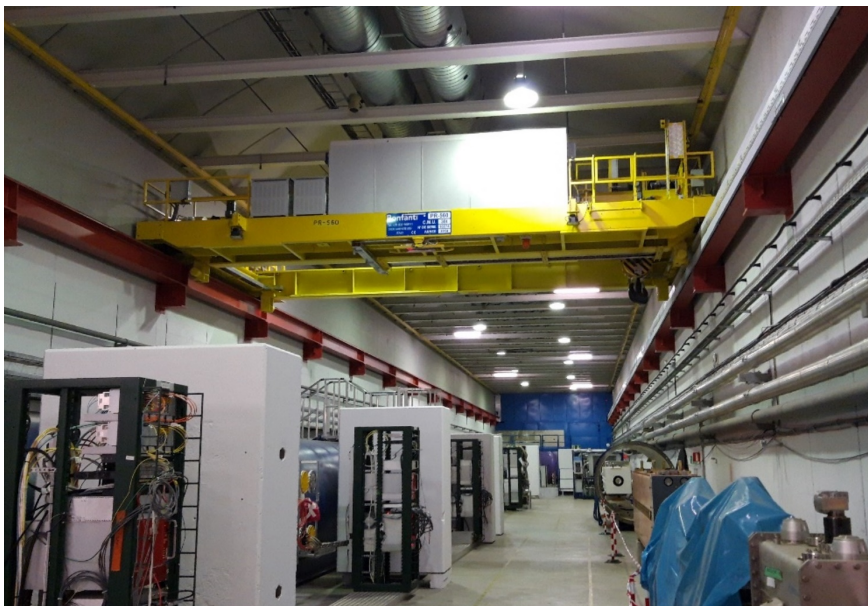
Figure 2 – The crane currently installed in TCC8
