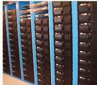
Tib Calorimeter Read-Out Subsystems installation
