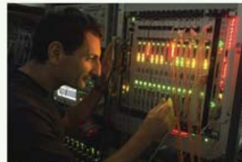
Working on Trigger components
