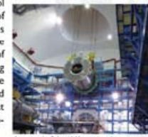
Lowering the Solenoid Magnet into the cavern
