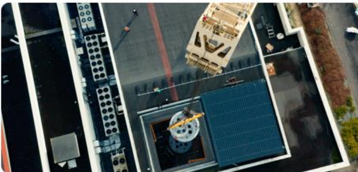
Bunker ceiling open for the installation of the C400 in 2024
