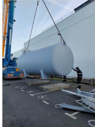
Quench tanks for He recovery
