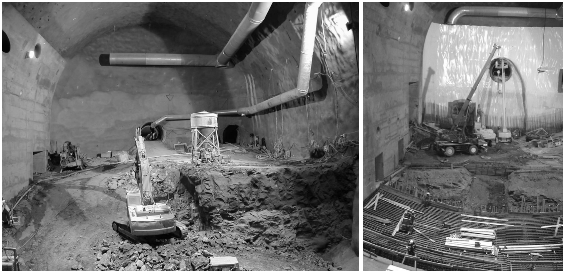
Figures 9 & 10 – Construction of experimental cavern UXC 55
