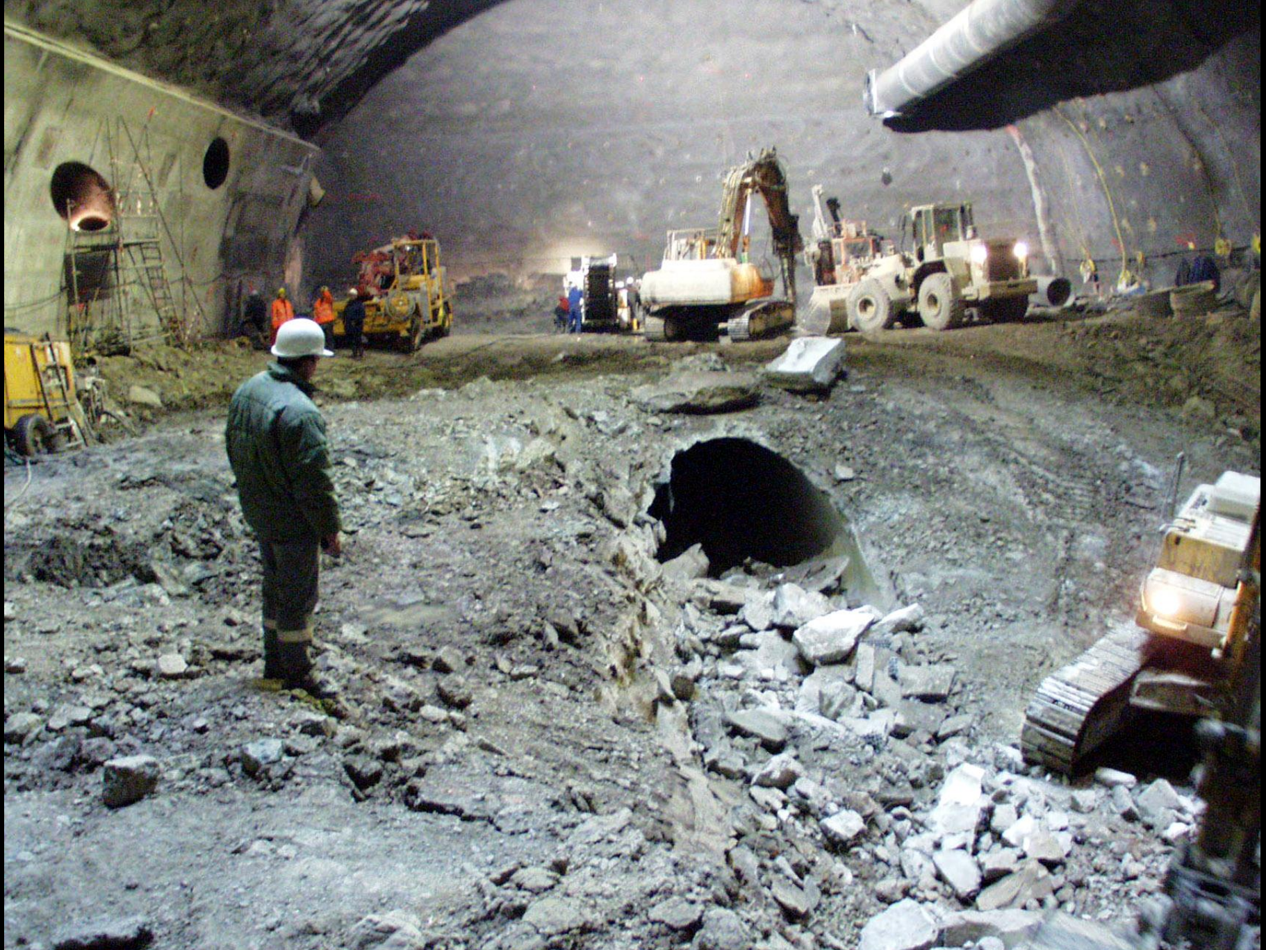
Point 5 - UXC55 cavern excavation - LEP demolition - January 23, 2002 - CERN ST-CE
