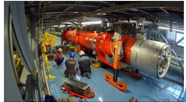
First magnet installation (Q2a) into the IT String at CERN
