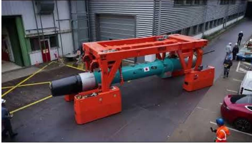
Installation of the D1 magnet into the IT String at CERN
