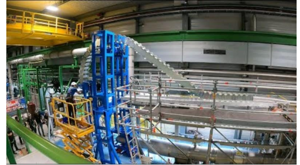
Installation of the Cold Powering System into the HL-LHC IT String
