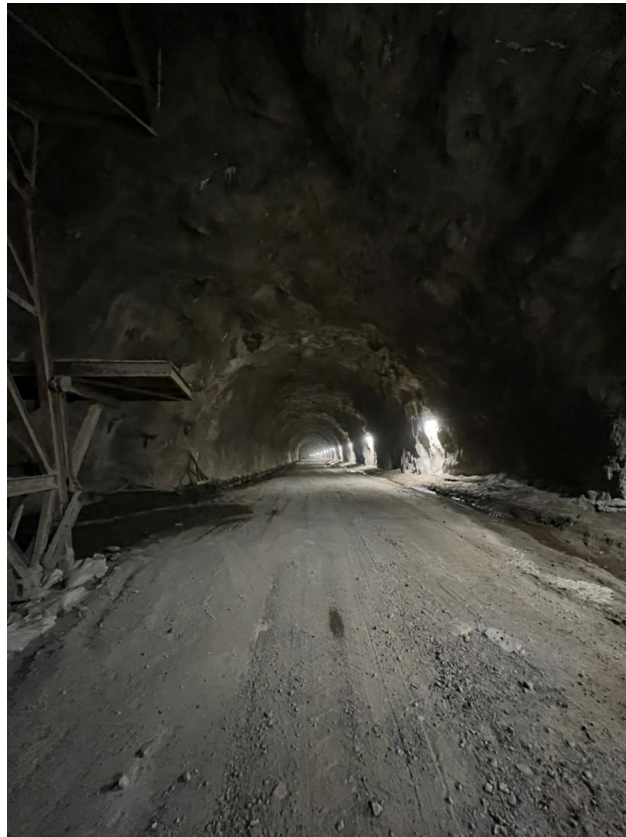
Figure 17-2: Inside the Huguenot Tunnel. Photo credit: courtesy JJ Van Zyl/Stellenbosch University.
