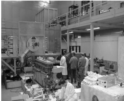
The Russian 100 J, 1 Hz CO 2 Laser Amplifier in building 363 (“Faraday Cage”), being commissioned
