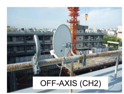
We used the Ku-band antennas with LNBF (for circular polarization), which is CBS45AST by Nippon Antenna, which has 45 cm diameter, the received frequency of 11.7-12.75 GHz and the converter output frequency of 1032-2072 MHz. We use two sets of antenna+LNBF pointing to different directions.
