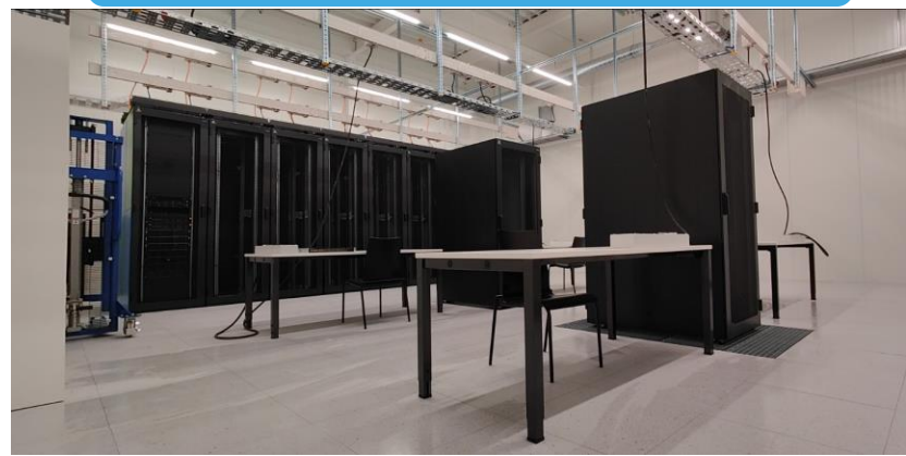
Racks with air/water passive cooling
