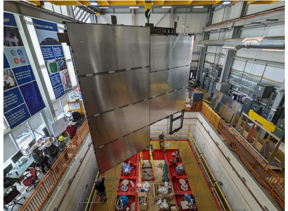
The first wall of the Cosmic Ray Tagger (CRT), consisting of individual scintillating strip modules being installed on the downstream end of the cryostat.
