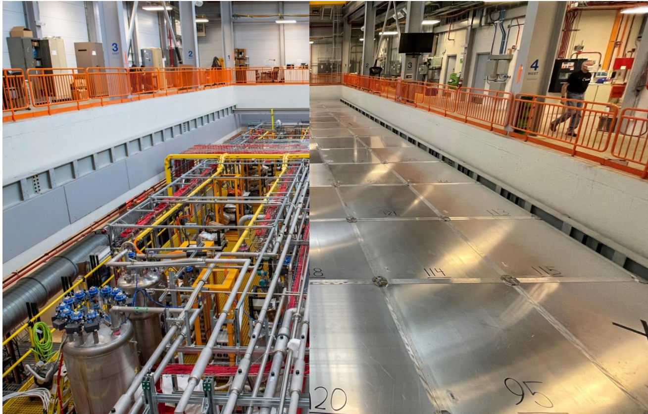
Before and after the Top CRT installation
