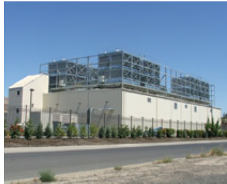
Google's data center at the Dalles on the Columbia river
