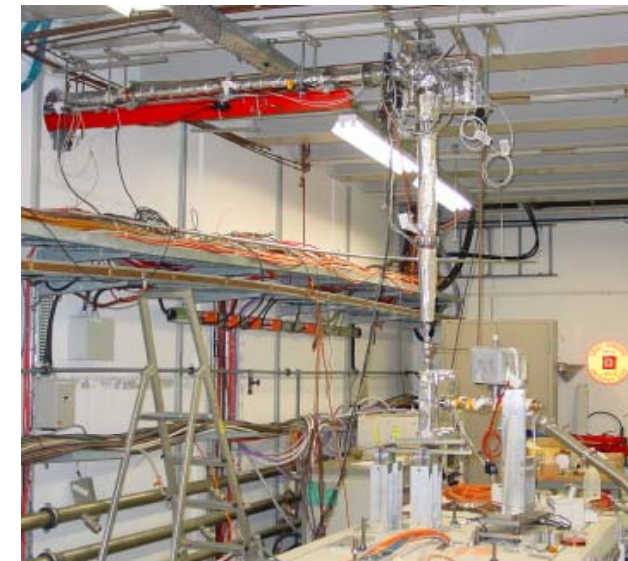
high power load / accel. structure
