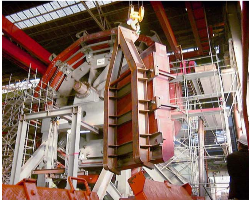
Pre-assembly at Deggendorf (1999)
