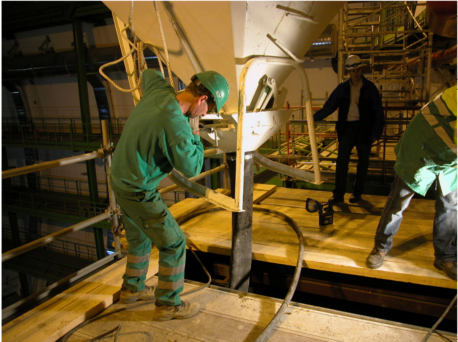
Concreting of blockhouses May 2006
