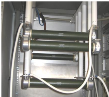
38 kV PSU – resistor bank
