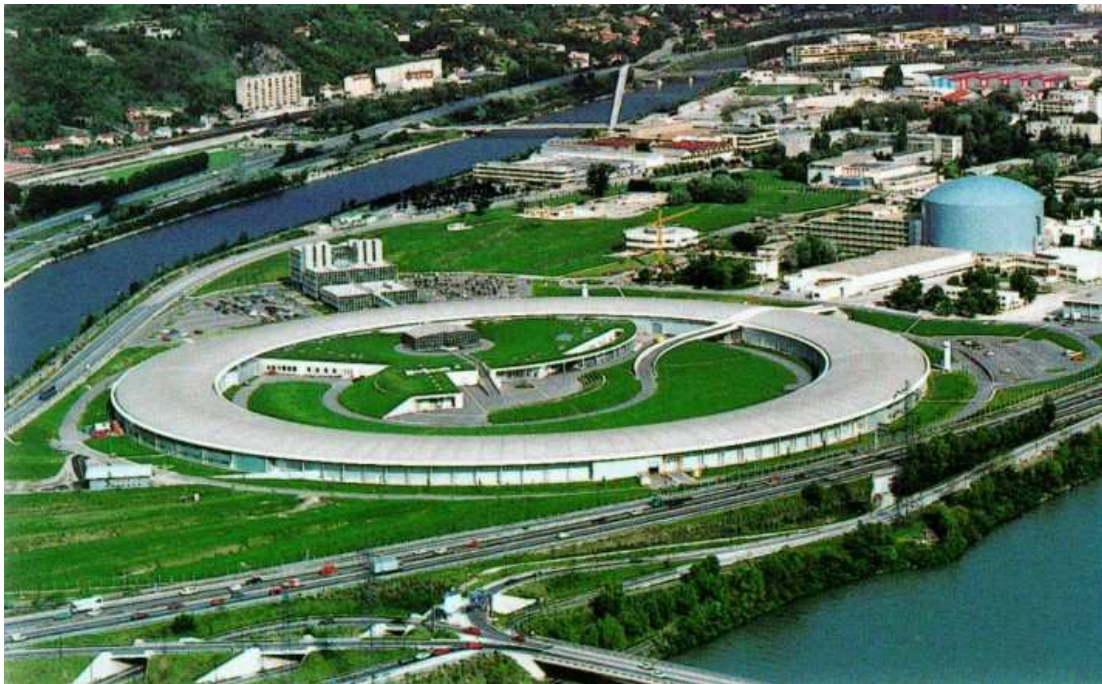
Fig. 6.3 Site of the European Synchrotron Radiation Facility ESRF in Grenoble
