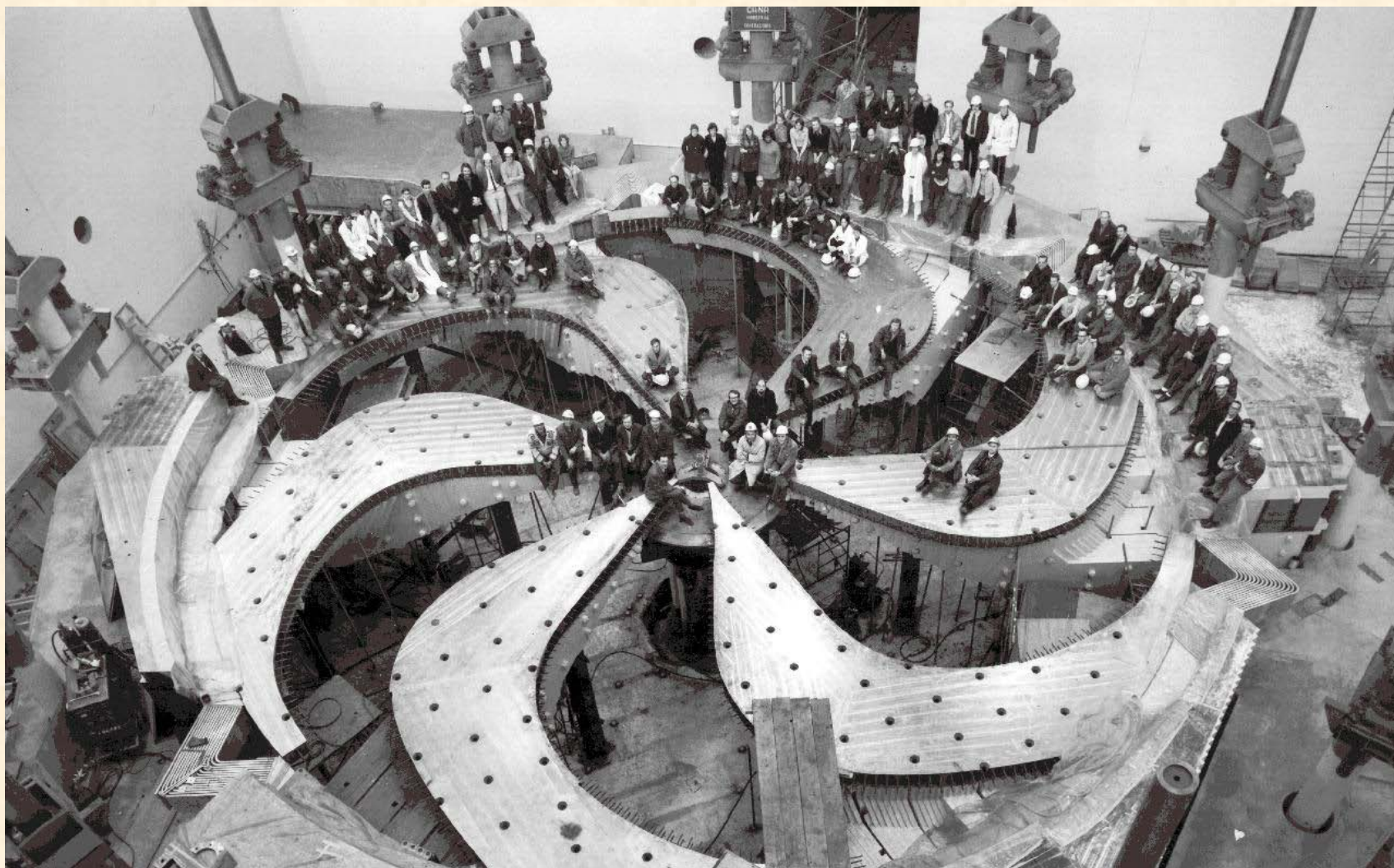
Lower half of the Main Magnet poles
