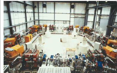
Example: heavy ion storage ring TSR 8 dipole magnets of equal bending strength
