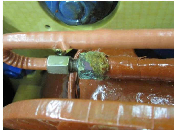
Degraded hydraulic connection brazed joints
