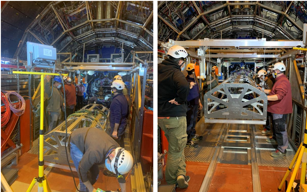
OB Top chassis for extraction (ALIITSUP0957) before (Left) and after (Right) to be lifted by the manual lifting device (ALIITSUP0848).
